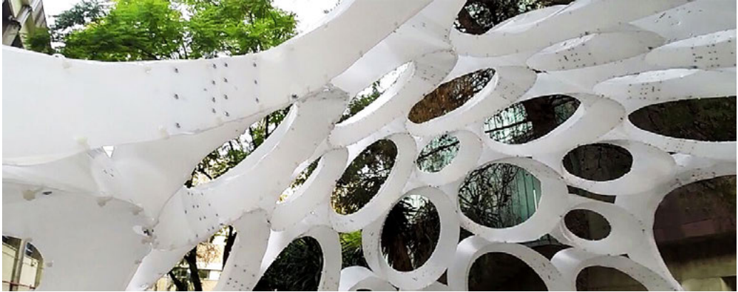
Figure 1. Photograph from the interior of the Archimedean Pavilion prototype, composed of inclined rotational parabolic domes materialised with lightweight conical components.
