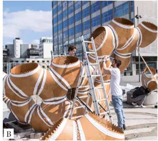
Figure 1b. The double-layered timber segments are most visible during the demonstrator's construction phase.
