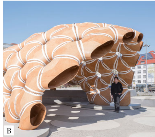
Figure 2b. The principle constructional morphology of such structures is transferred into a segmented timber shell construction system with bent plywood strips.
