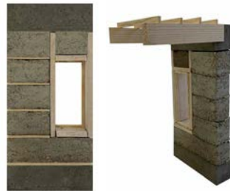
Constructive Picture of the window module
