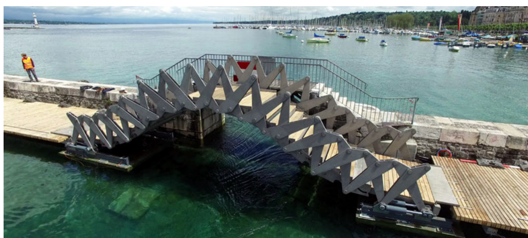
Figure 19. The footbridge in situ during the rise. The movement from flat to raised takes around 90 s.
