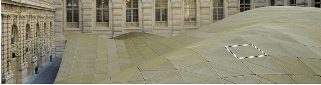
Figure 1. Non-smoothness from geometric constraints: The Cour Visconti roof in the Louvre is a hybrid mesh consisting of both triangular and quadrilateral glass panels, for reasons of efficiency and weight optimisation. The triangle mesh originally intended by the architect is achieved by placing triangular shading elements on top of each panel. Merging of two triangular faces into a quad consumes one degree of freedom, so this mesh is not as optimally smooth as would have been possible with a triangle mesh.
