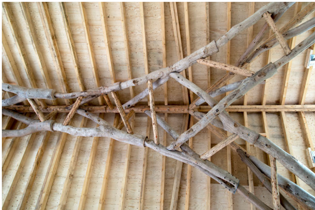
Figure 13. The structure fully loaded with its roof added. The complex form of the truss contrasts with the regular lines of the roof above. Image: Valerie Bennett.
