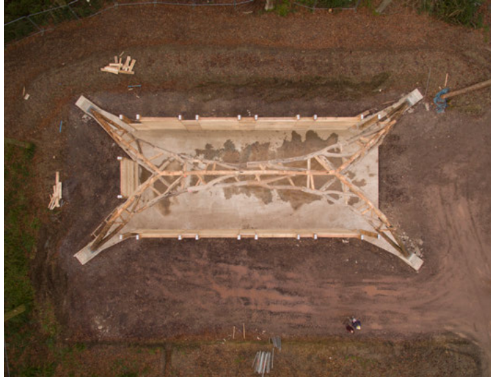
Figure 12. A drone photo of the Wood Chip Barn's primary structure erected on site. Spanning 25 m from front to back and 10 m side to side, the arching truss rises to 8.5 m at its zenith.
