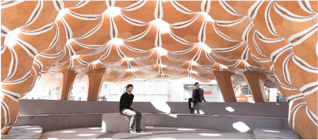
Figure 10. Photograph of the demonstrator. Once assembled, the robotically sewn segments act together as a rigid, double-layered shell.
