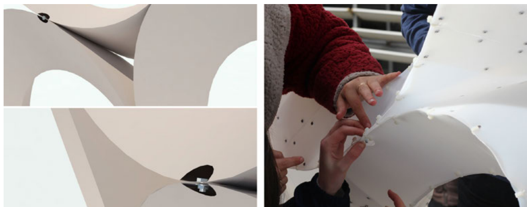
Figure 9. Two pictures and a photograph of the connections between components, including the drilling for the screw and the opening to operate on it.
