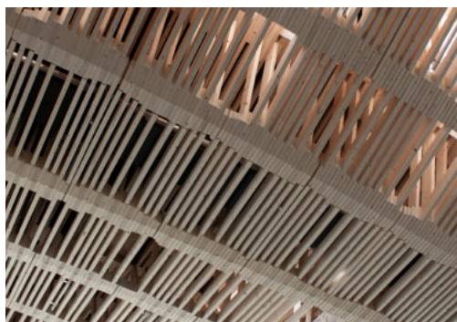
Figure 22. Detail soffit view of the completed roof. The varying width of the diagonal slats manifests itself in the connections. The shadow gaps between the timber trusses allow for building tolerances and shrinking and swelling of wood.
