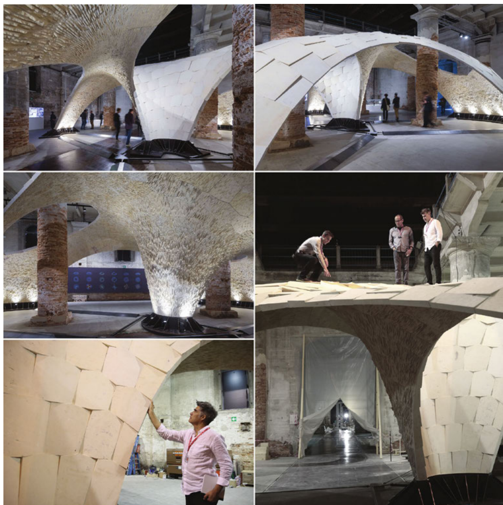
Figure 11. Finished cut-stone vault in the Corderie dell'Arsenale of the Architecture Biennale in Venice.
