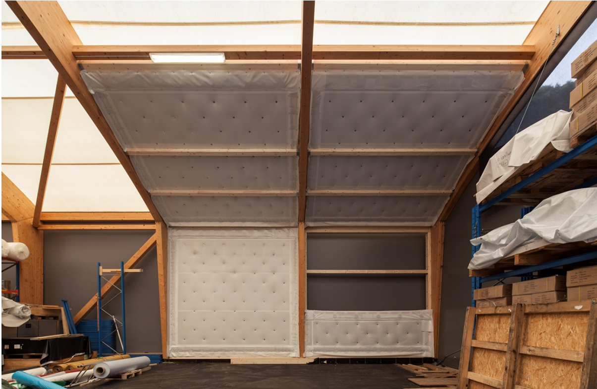
Fig. 2: Prototype of the textile retrofit system.
