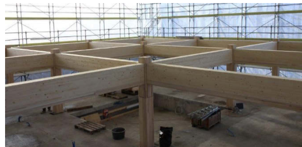
Fig. 1: Post-tensioned timber frame.
