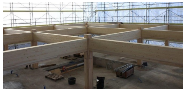
Fig. 1: Post-tensioned timber frame.
