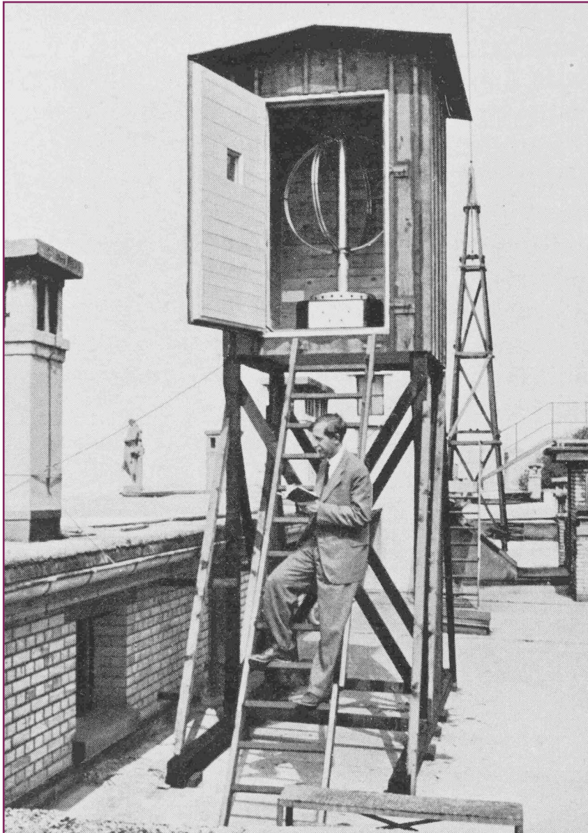
Figure 13.3: The radiogoniograph on the roof of the physics building of ETH around 1937; on the ladder stands Jean Lugeon, who became director of the Meteorologische Zentralanstalt in 1945. Note the (rotating) crossed loop antennae in the wooden hut. (Lugeon, 1939)
